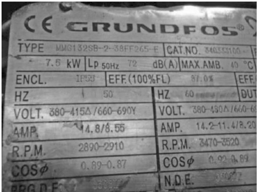
Figure 7-5 Motor nameplate
