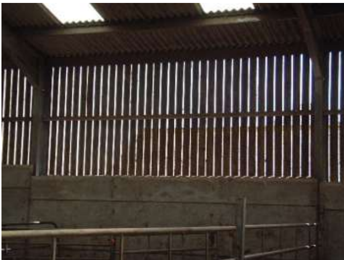
Plate 5 – space board for side ventilation.
