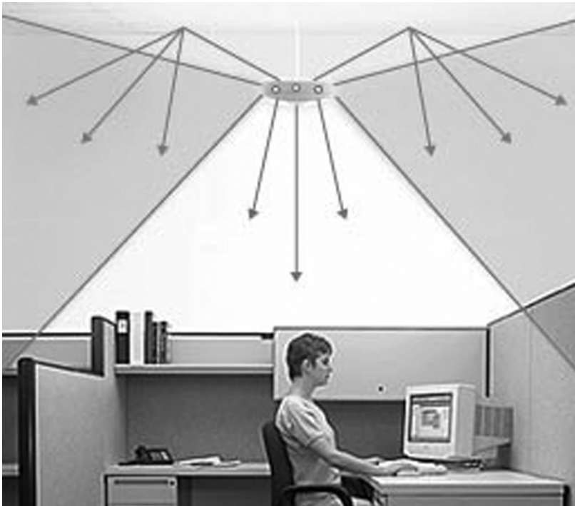
Figure 6-25 Up-Down Light Fixture
